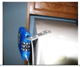
1. In this picture, a  $2^{"} \times \frac{1}{2} \times \frac{1}{8}$  flat mending strip was screwed into existing screw hole on top of the refrigerator. These holes are also found in the space between the upper and lower compartments on the refrigerator. These holes are normally used to reverse the direction a refrigerator door opens. You simply remove the plastic cap that covers the hole and screw on the strip.
